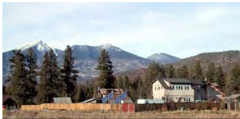
Figure 2 - Trust Headquarters (Note the solar panels)
